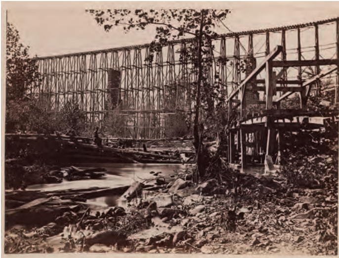
Sherman’s March No. 4 - Trestle Bridge at Whiteside - Racoon Mountain, TN
