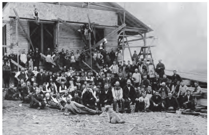
Construction of Iron Pier in 1890
