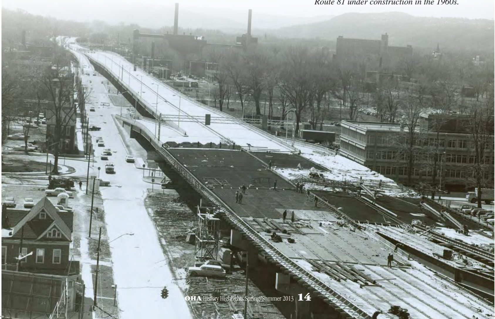
Route 81 under construction in the 1960s.
